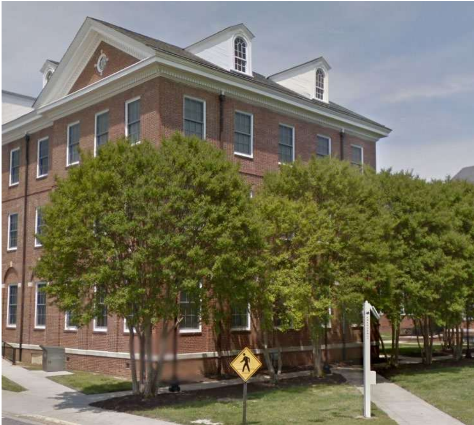
South Elevation, looking from Hayden Drive
