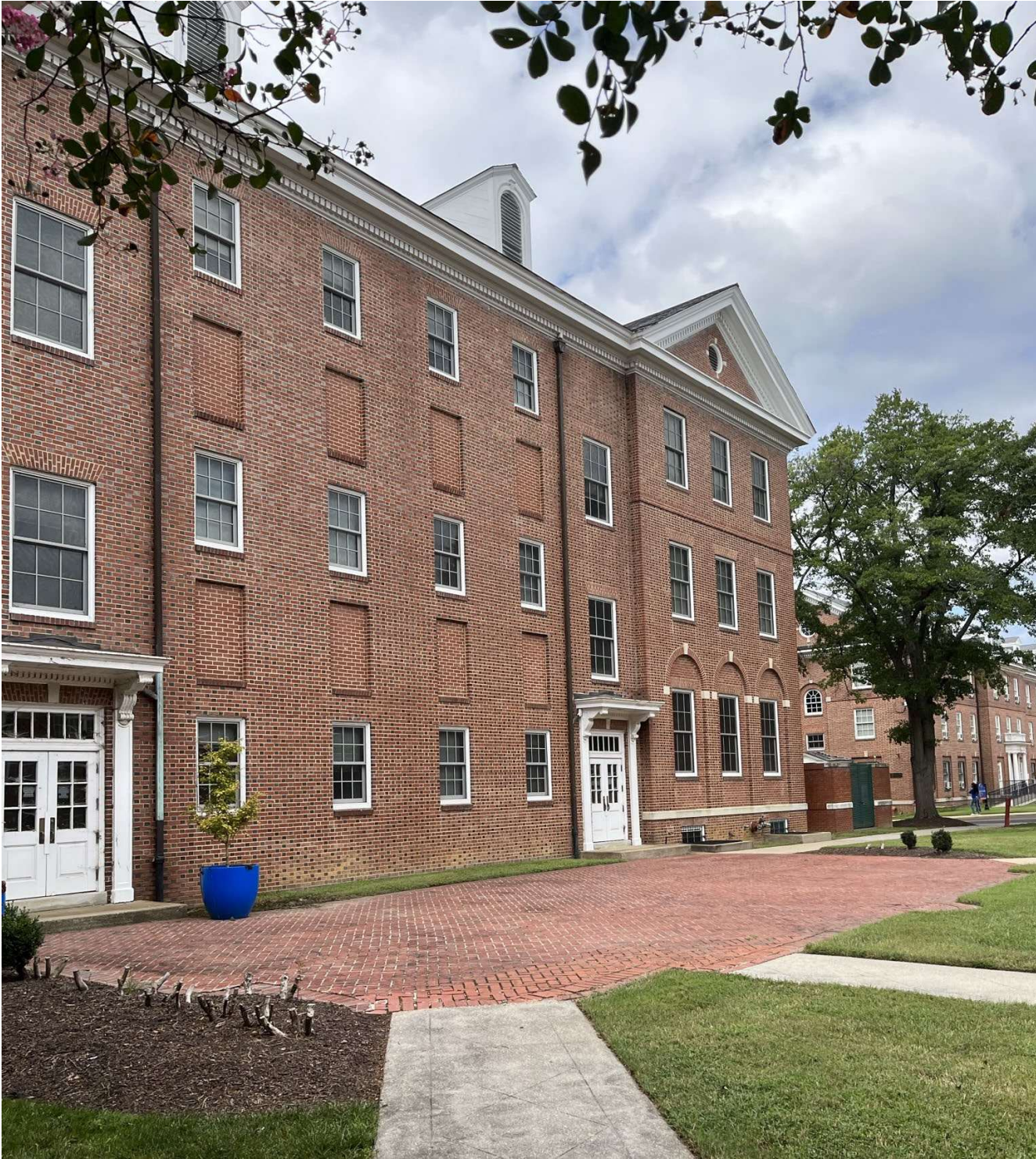
East Elevation, standing from the path
