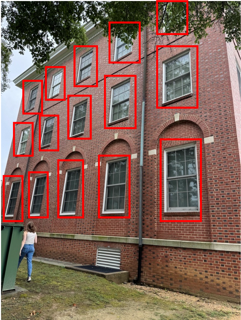
Right Basement Window In View
